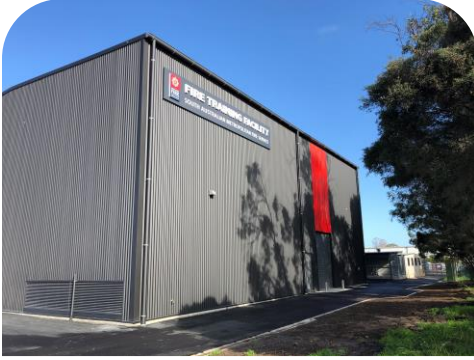
Above: MFS Angle Park Structural Firefighting Training Facility.
